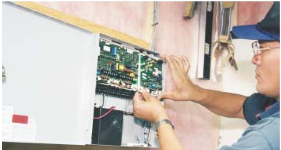
The installer snaps in a radio receiver to give users simple Keychain Touchpad control and the flexibility to install wireless or hardwire sensors.
